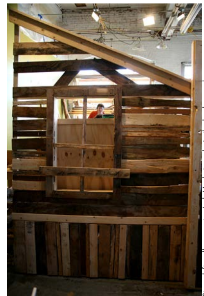
Stage left wall; carpenter Josh Hackett works in the background
